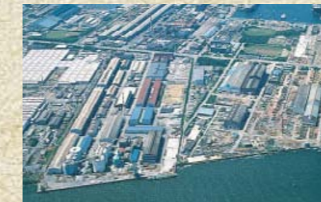
⑪ Chiba Plant
