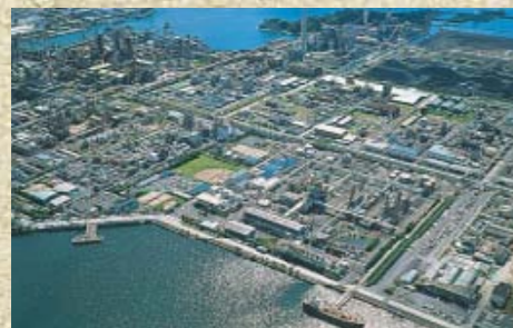
③ Tokuyama Plant
