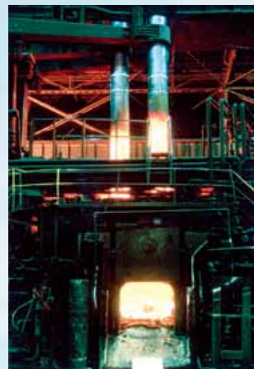
Graphite electrodes being used in an electric arc furnace
