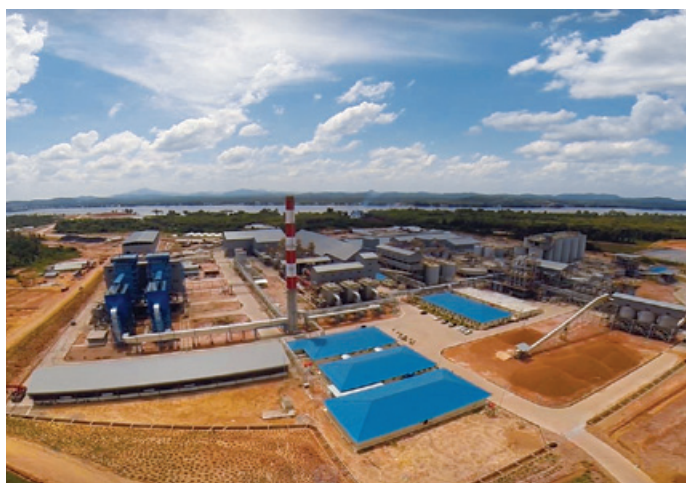
PT. Indonesia Chemical Alumina's new plant
